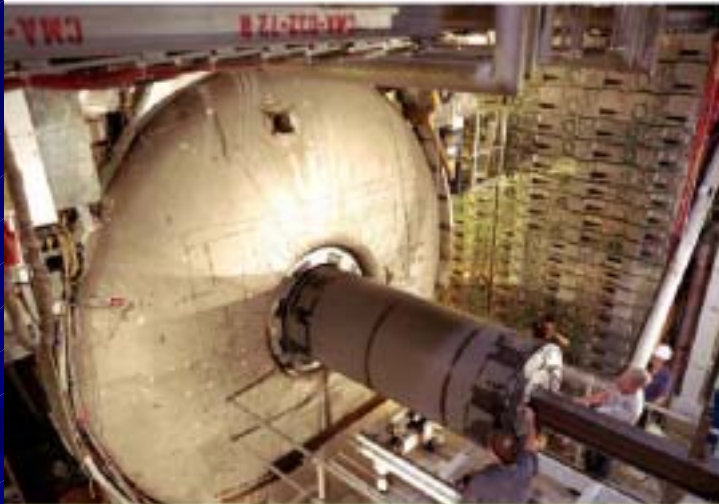
DØ fiber tracker installation
