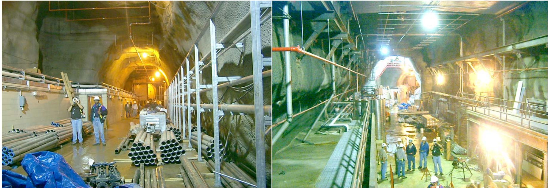
MINOS Access Tunnel (left) looking upstream MINOS Hall (right) looking upstream
