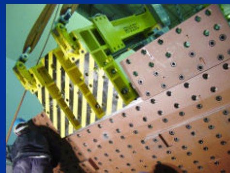
33mm diameter pins in the connecting plates between modules carry the tension load below the saddles which resists the moment from the modules above the saddles
