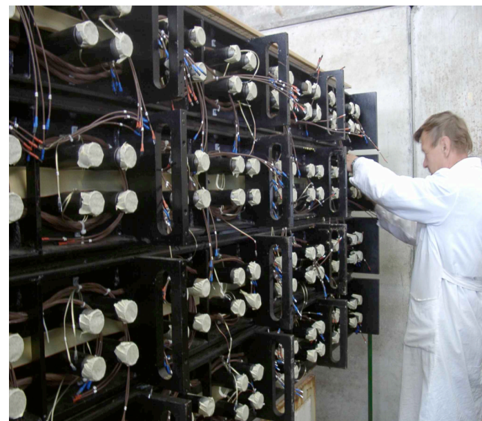
All H-cal module completed
